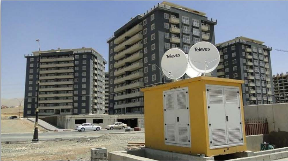
Prefabricated Concrete Substation 11/24/36 kV
